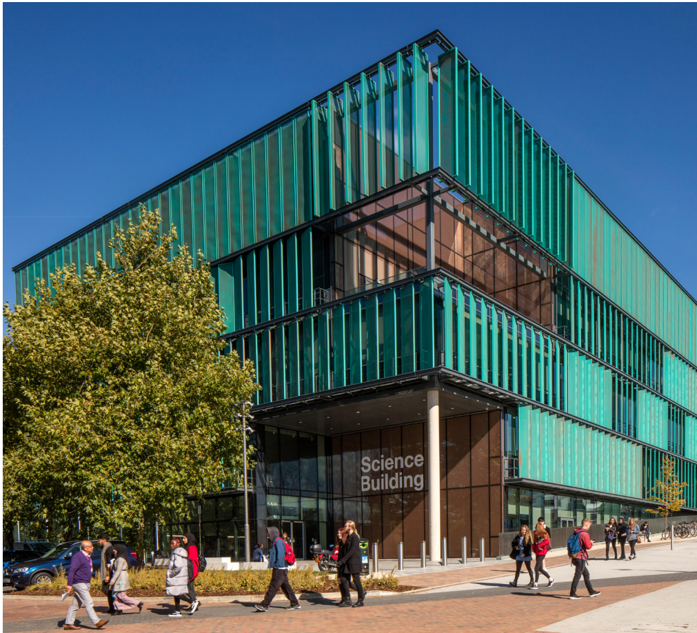
Science Building, College Lane Campus
